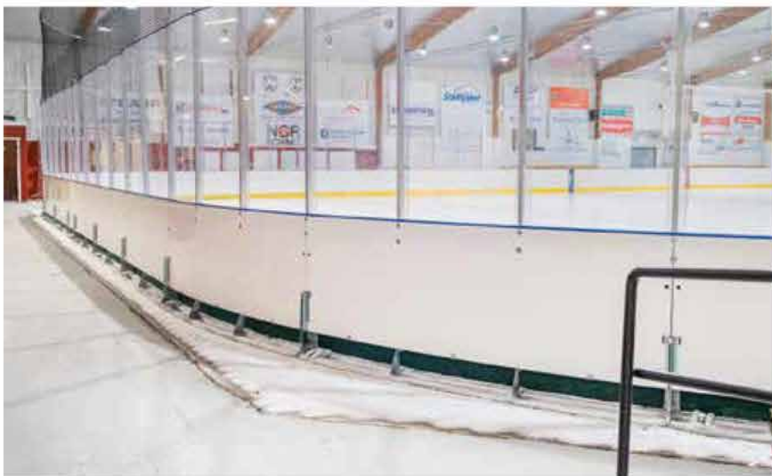
Installation into ice with steel plates
