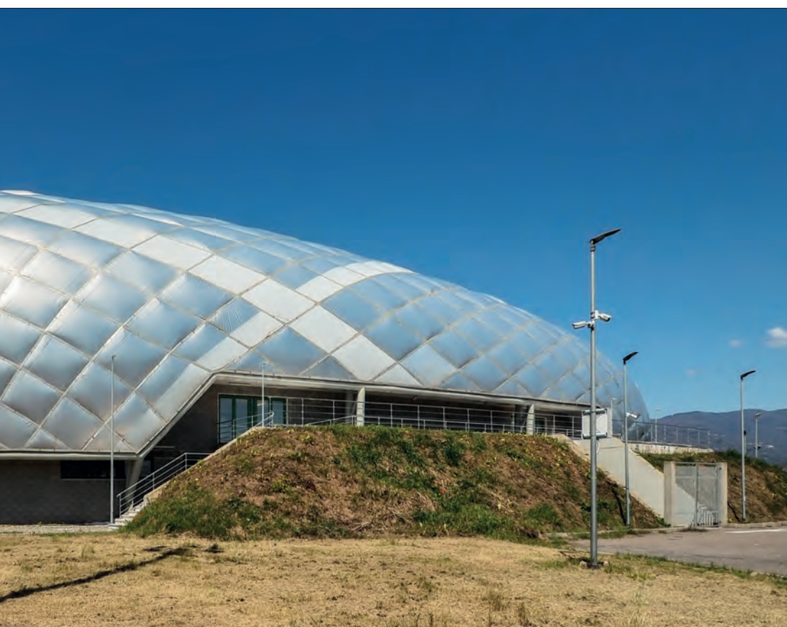
In the photos, two views of the interior and two of the exterior, with a detail of the ETFE shell.
