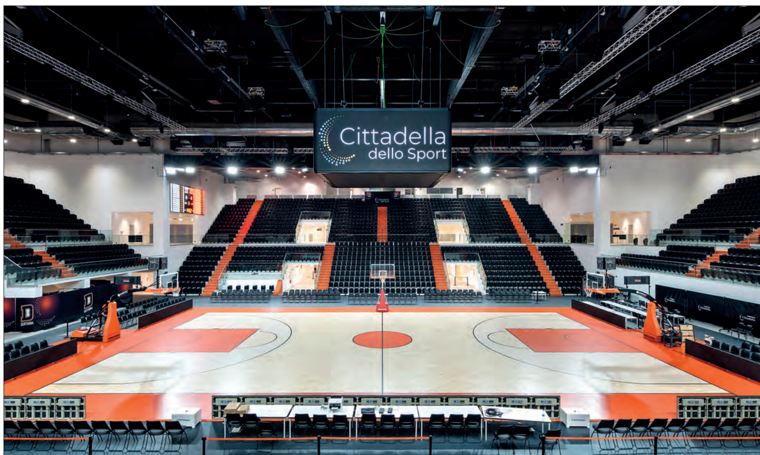
On these two pages, the sports hall. At the top, plans of the ground floor and upper floor. Below left, view of the interior with the glass balustrade (photo: BG / Tsport), on the side, section showing two types of balustrade attachment. On the right, overview of the interior.
