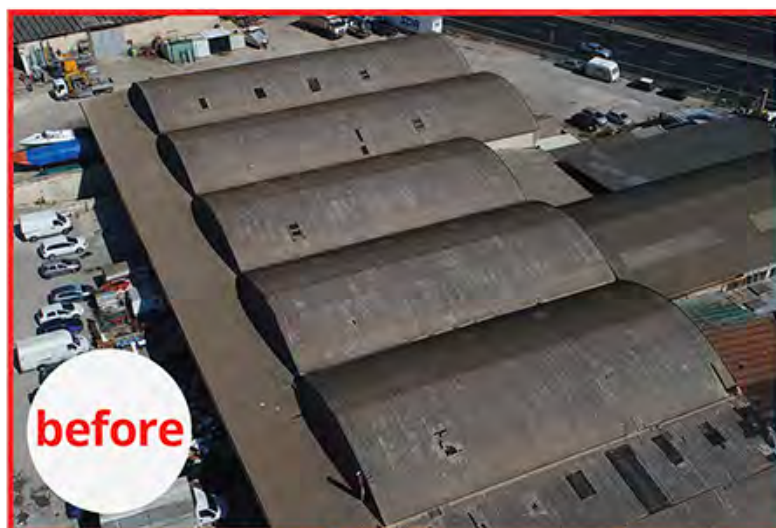
Eternit or cement-asbestos roofing
